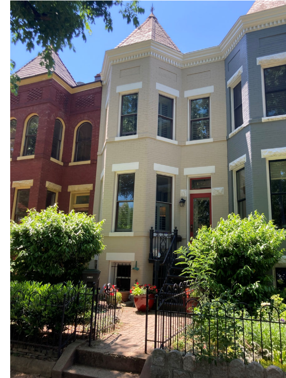
EXISTING FRONT FACADE
